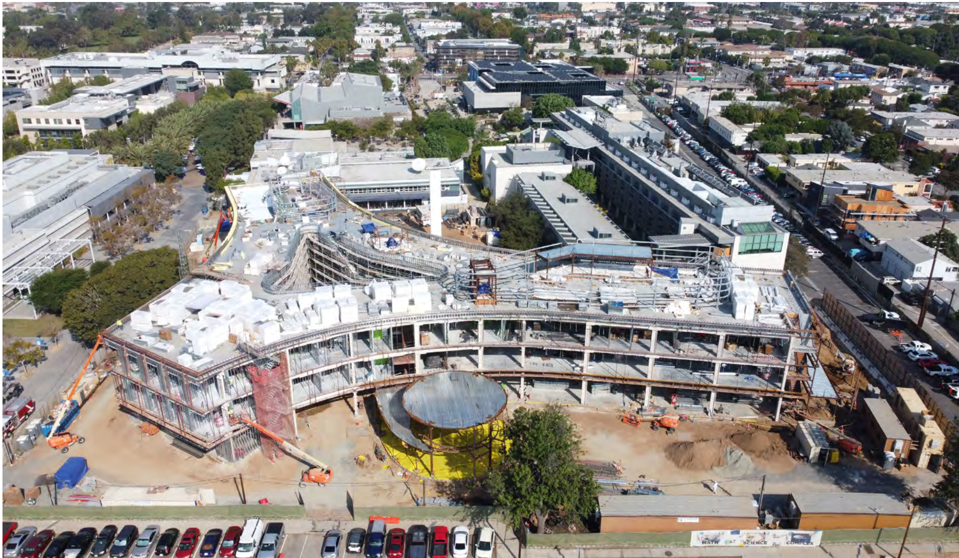
Math and Science building construction
