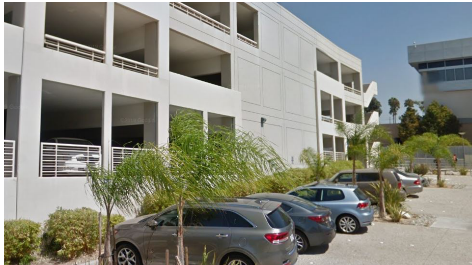
EV Parking in SMC underground garage
