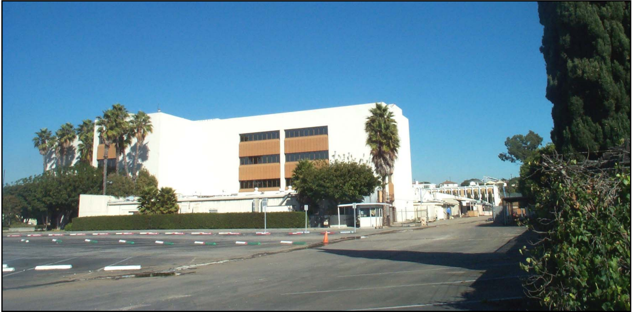
VIEW FROM SOUTHWEST CORNER OF PARKING LOT
